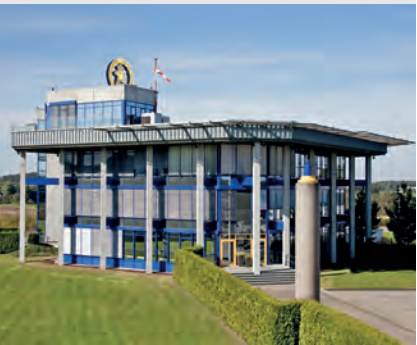
Joh. Clouth GmbH, Hückeswagen, Germany Head office of the Clouth Group
